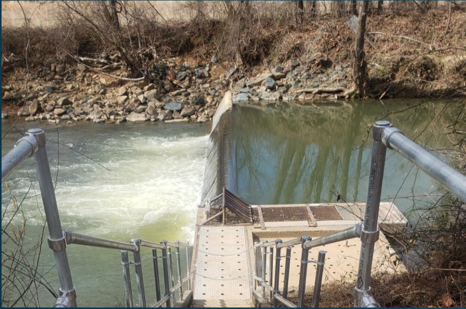
North Rivanna Low Head Dam
